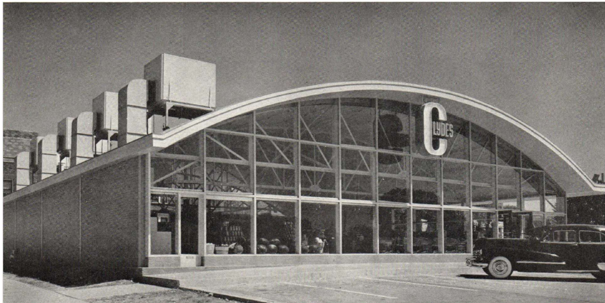
Figure 4. Photo c. 1949 showing the large air conditioning units visible on the north roofline, wood framed glass wall, and exposed bow truss structure of Clyde's Supermarket. [Source: Progressive Architecture , May 1949, 73.]
